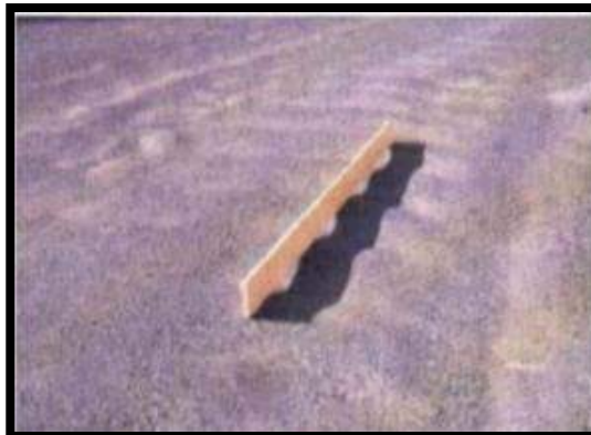
Gambar 2.25 Keriting/Bergelombang ( Corrugation )
